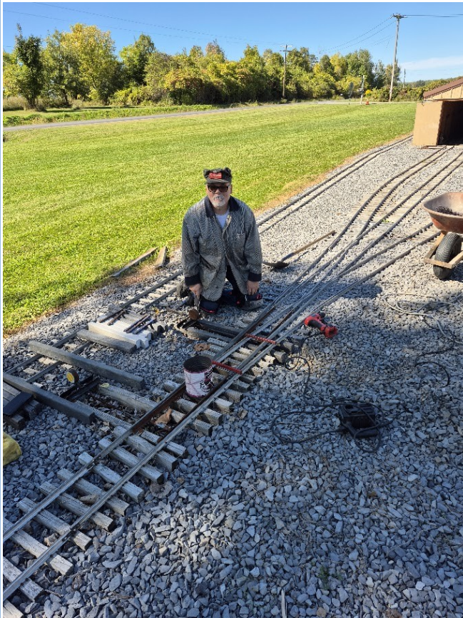
Don Jermyn is replacing the old wood ties in front of the club's car barn, with long-lasting plastic ties. He is starting with the switch ties.
